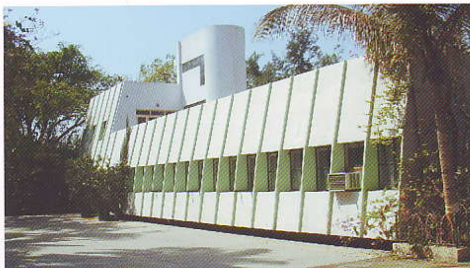
Administrative office within the plant
